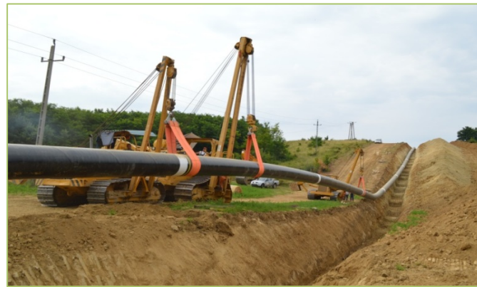
Some parts under construction
